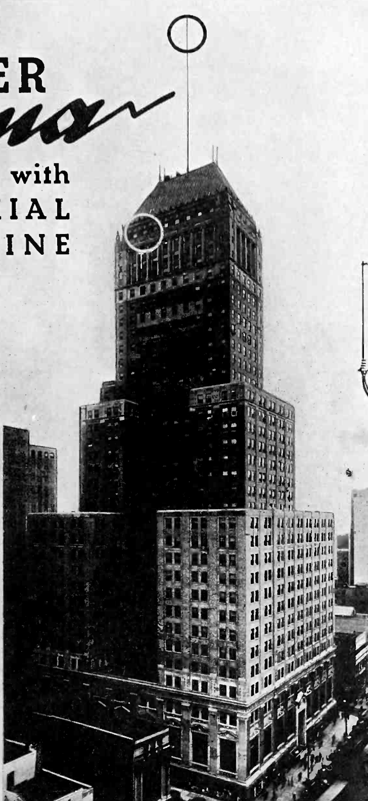
National Newark and Essex Bank Building, Showing location of transmitter and antenna connected by ISOLANTITE COAXIAL TRANSMISSION LINE.
